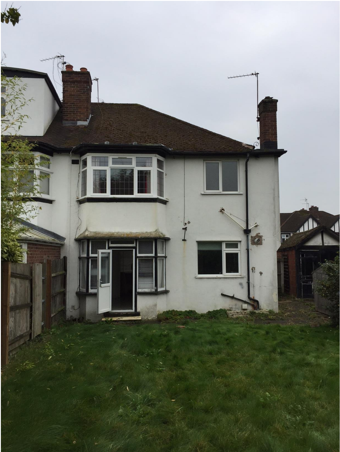
Rear elevation of 11 Sherington Avenue
