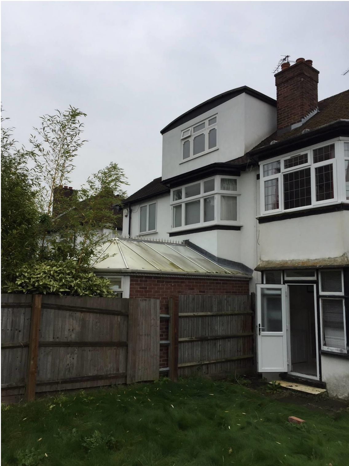
Rear elevation of the adjoining property No.15 Sherington Avenue
